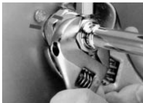
Rotate Swivel Nut ¼ Turn More
